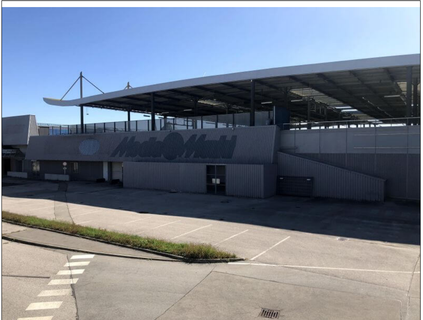
Leerstehendes Shopping-Center, (c) Mathias Sander
